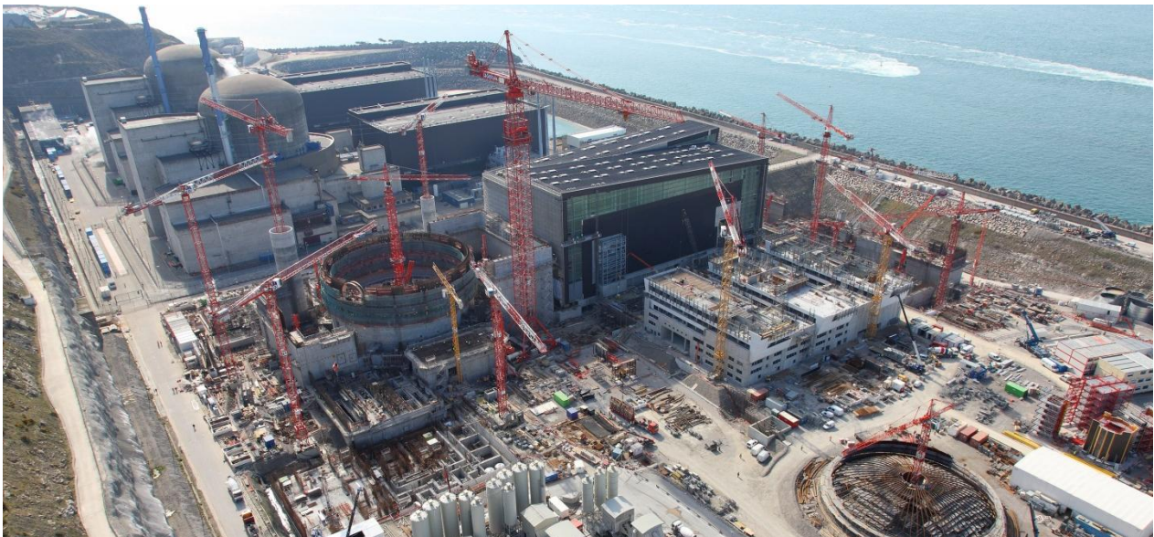
Flammanville 3 under construction © EDF 2010.
