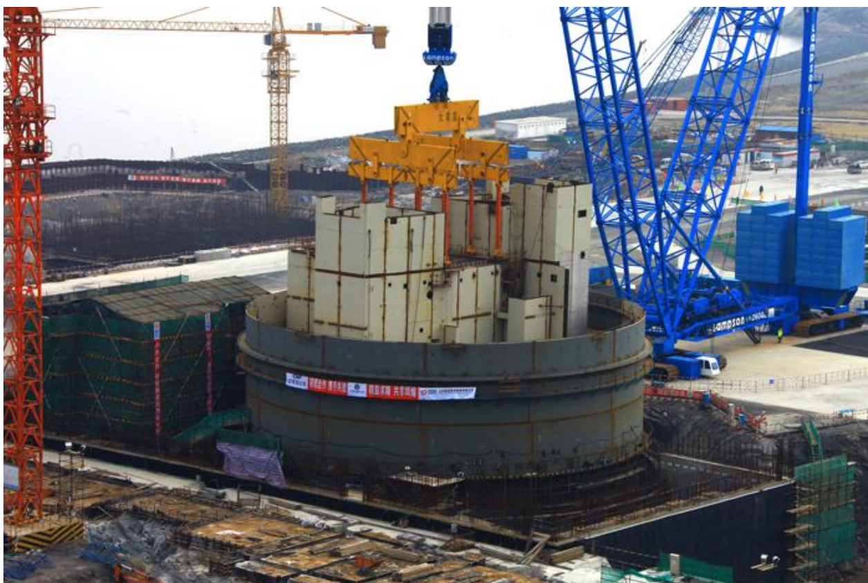
AP1000 under construction, Sanmen, China; © SNMPC 2010.
