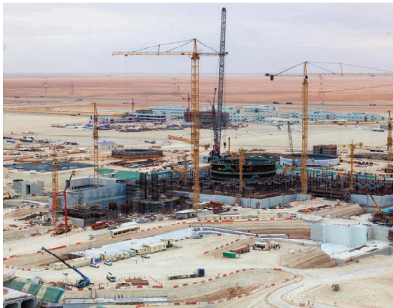
Barakah site—APR1400, United Arab Emirates, April 2013 (ENEC).
