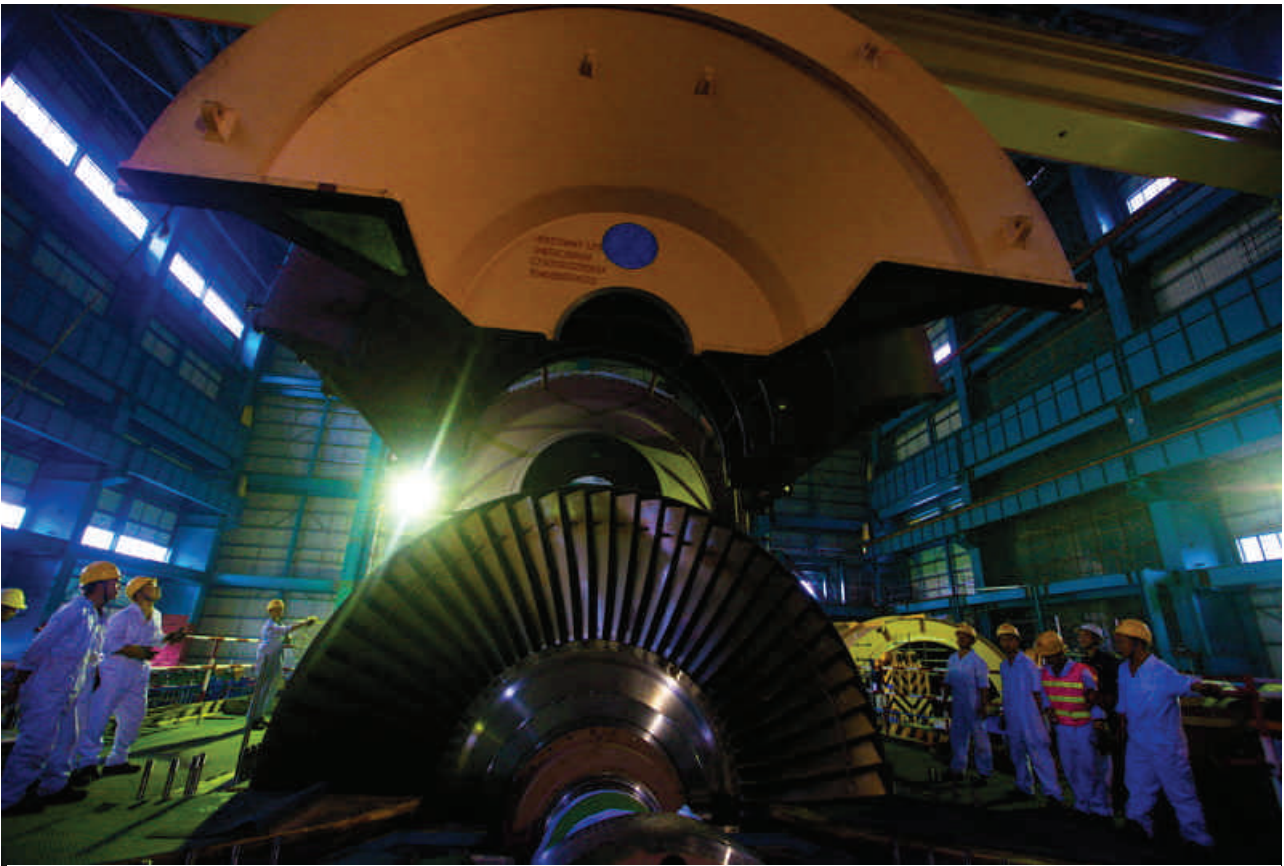
Taishan Unit 1—Turbine installation, EPR, China, October 2013.
