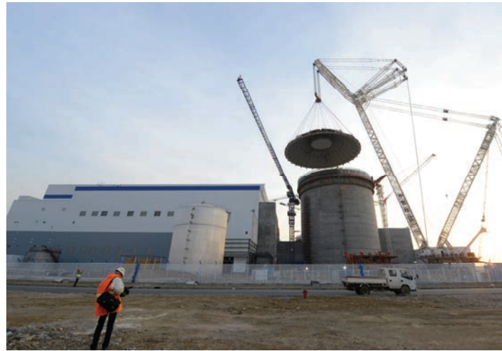
Haiyang Unit 1—Dome Installation, AP1000, People's Republic of China, December 2013.
