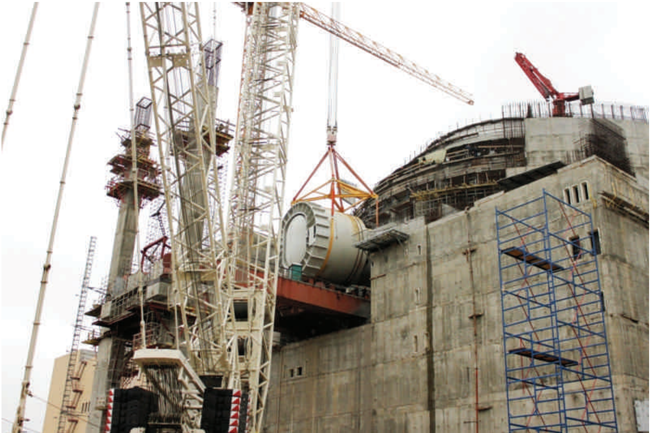
Novovoronezh II—Gateway installation, VVER, Russian Federation, November 2013 (Rosatom).
