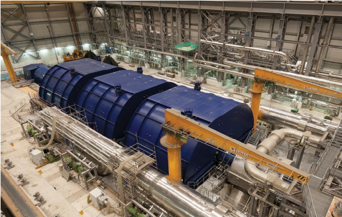
Olkiluoto Unit 3—Turbine island, EPR, Finland, June 2013 (TVO).
