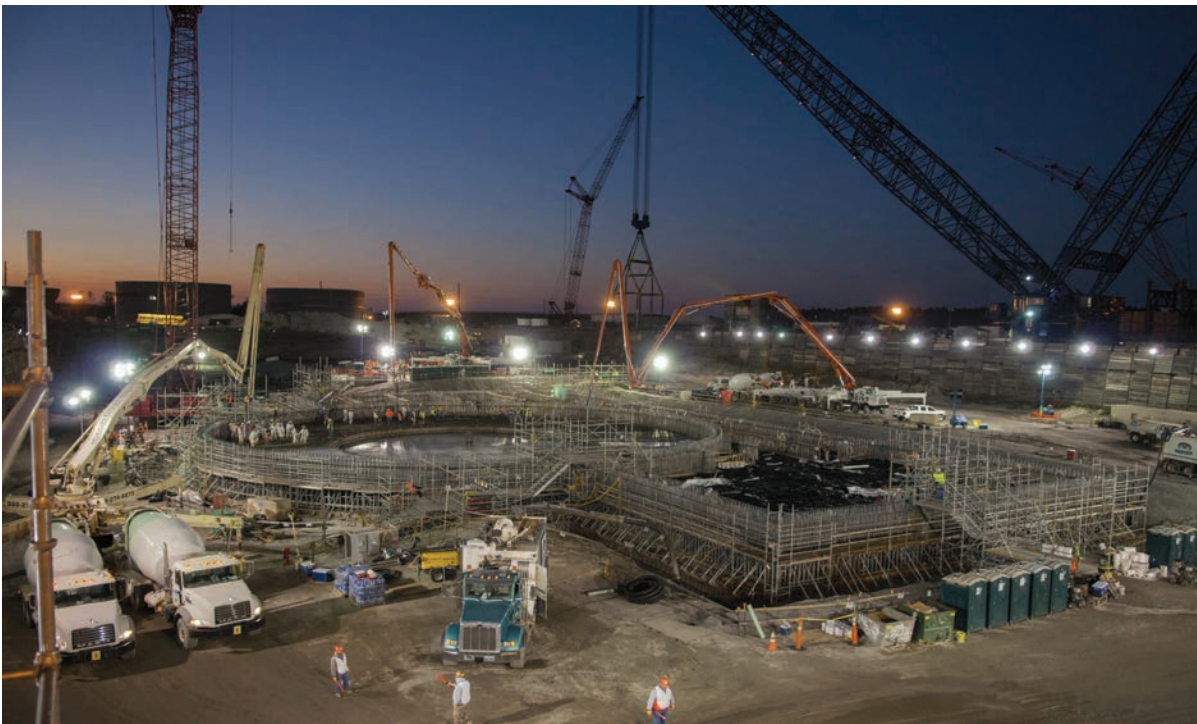
Summer Unit 3—Basemat concrete placement, AP1000, United States, November 2013 (SCANA).
