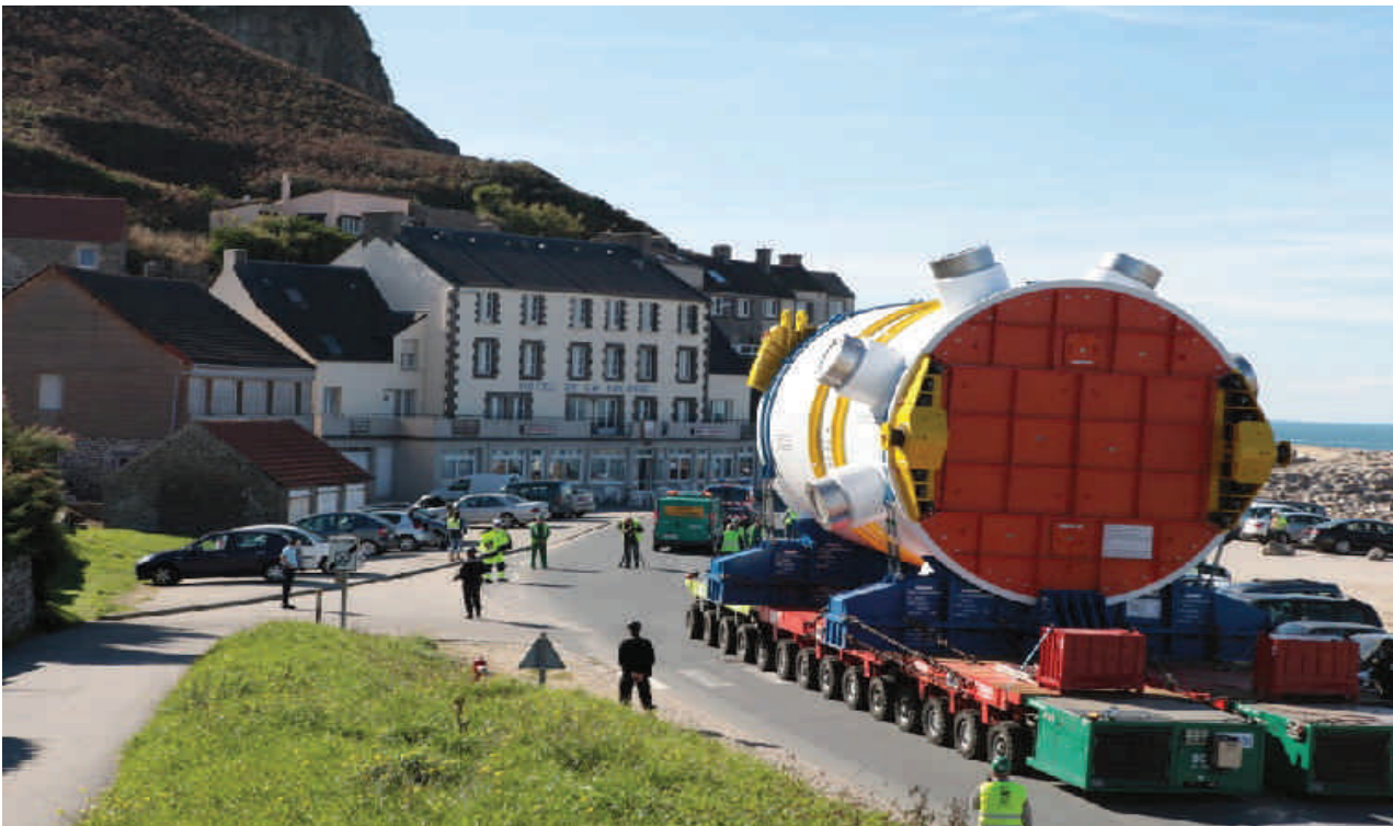
Flamanville Unit 3—Reactor vessel arrival, EPR, France, January 2014 (AREVA, DIKDAK).
