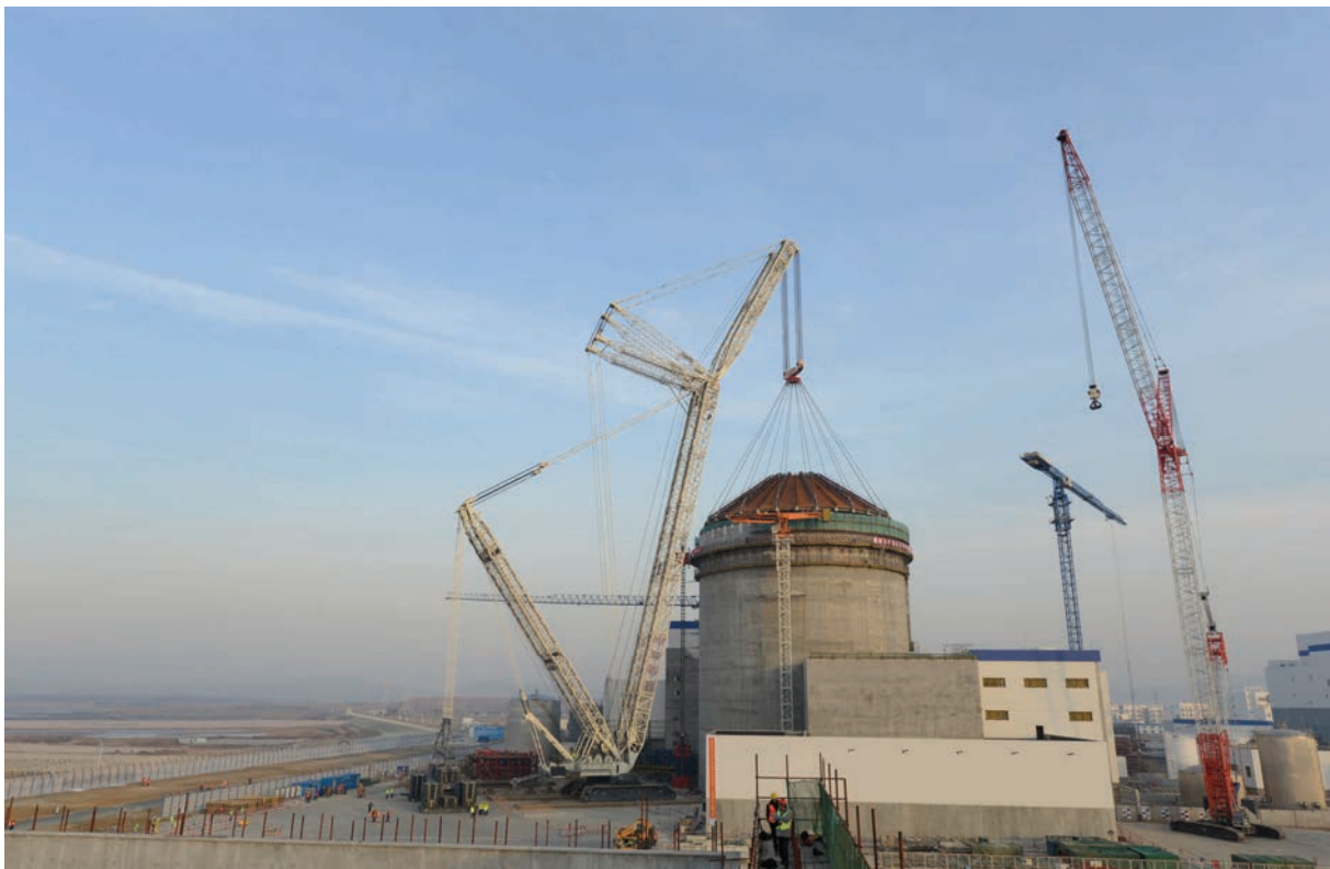
Haiyang Unit 1—Dome Installation, AP1000, People's Republic of China, December 2013.
