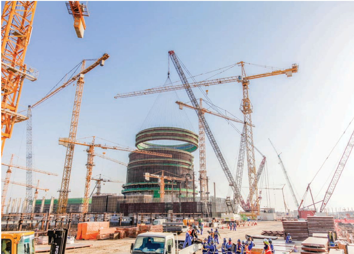
Barakah unit 1—CLP installation, APR1400, United Arab Emirates, November 2013 (ENEC).
