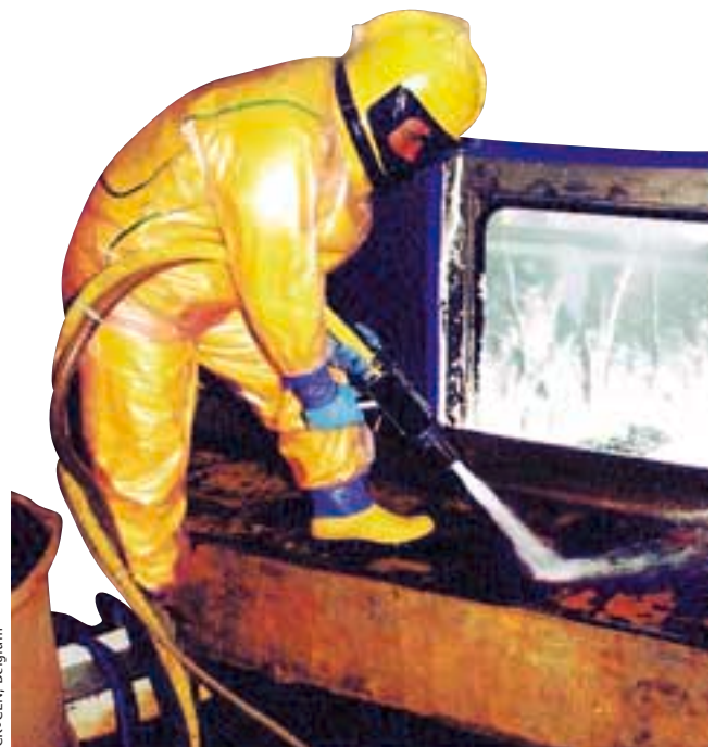
Decommissioning of large and heavy components by abrasive blasting.
