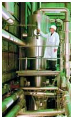
View of the PKL facility in Germany.
