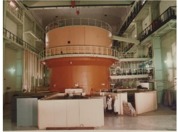
HWRR reactor hall
