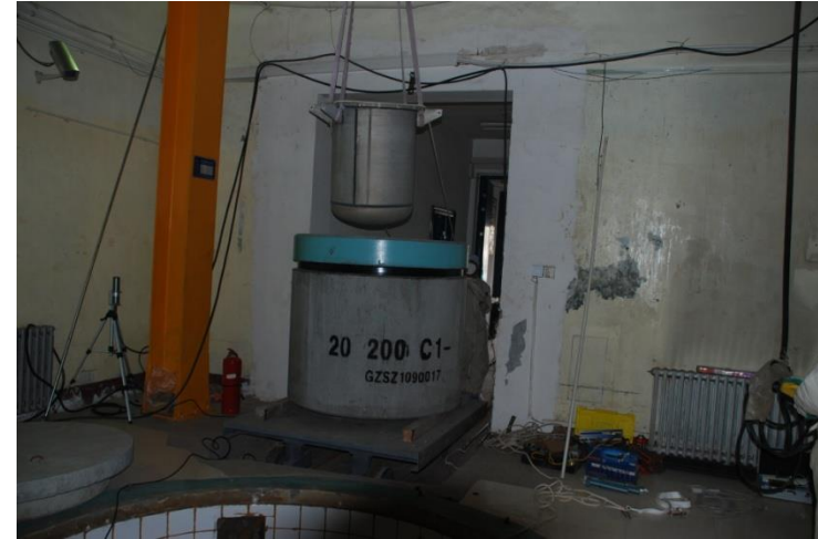
Hoisting lower cylinder to container after pool water discharge
