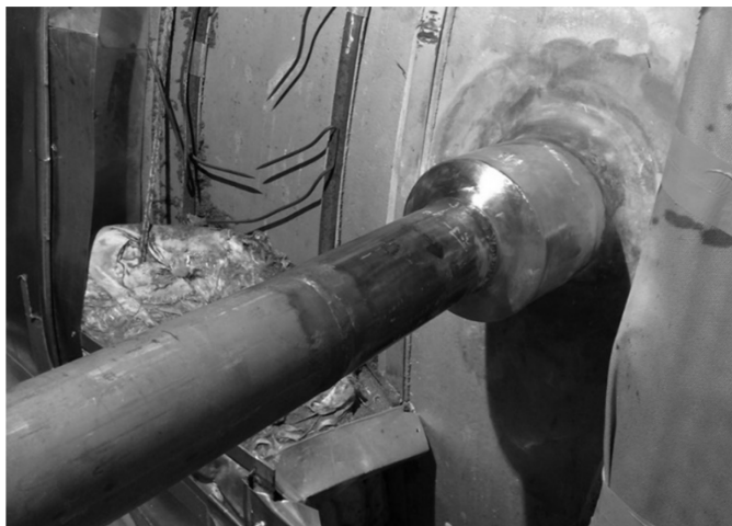
Figure 3-2: Dukovany-2 first-in-kind SEFW weld overlay
